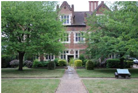
Having no stone in the area builders rendered brick to look like masonry
