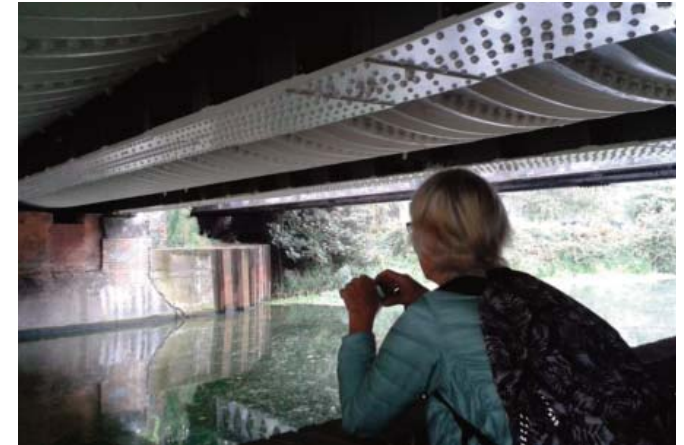
Pipes carrying waste from North-East London to Beckton Sewage Works. The route now known as the Greenway - pic by Jackie Morrison
