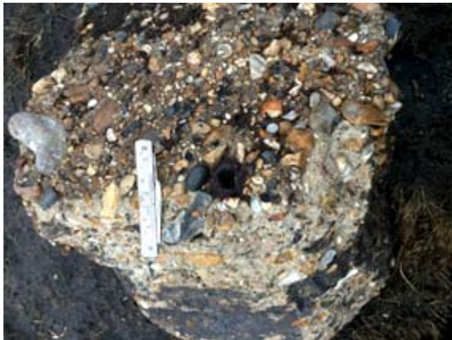
Another of the pudding bowl shaped objects though this one is more cylindrical, this time with the hole clearly shown, and the remains of a metal post of some sort (scale just over 3 inches). The rough nature of concrete also shown with pebbles from the flats possibly. Author photo.
