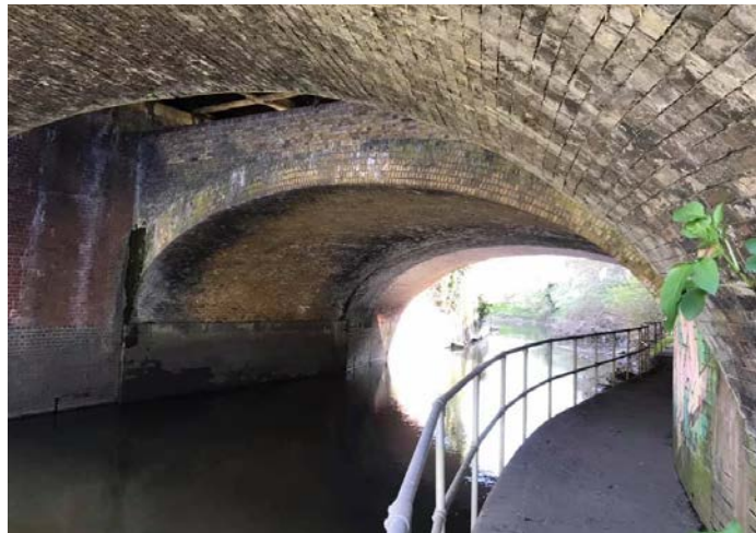
Railway crossing the Roding just beyond the North Circular - the bridge is actually about 5 different brick bridges built on top of each other.
