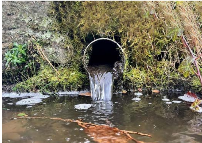
There are countless outlets into the River Roding. They are designed to take clean surface water from adjacent areas into the river and out to sea. However, under certain circumstances raw sewage and other pollutants can end up being discharged into our river. A problem that is becoming more and more frequent due to an ageing infrastructure and greater numbers of homes and other development.
