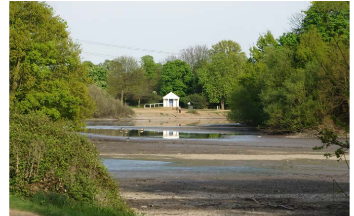
A V1 flying bomb is recorded as having hit the pond during WWII. This created a hole in the lining of the pond, and led to it leaking - adding to the recurring problem of water retention.
