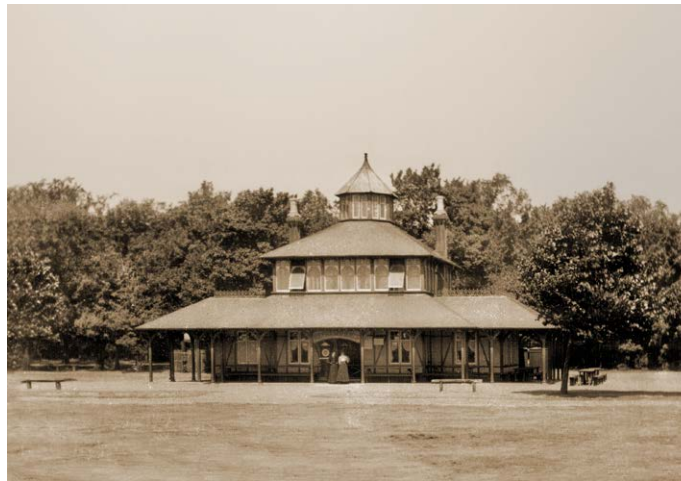
The Chalet in 1908. The Chalet was built in 1883 (the year after the Park was opened by the City of London) to serve refreshments. The Chalet burned down in 1948. The trees behind the site of the Chalet is named Chalet Wood, which is now well known for the display of bluebells in the springtime.
