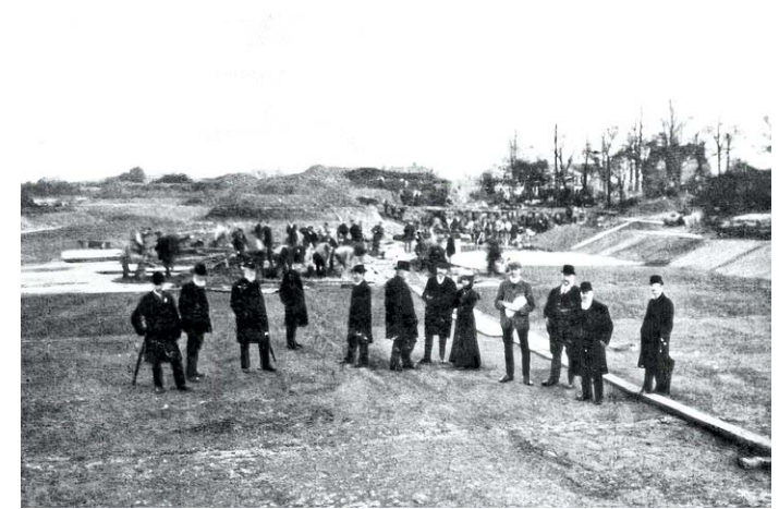
Members of the West Ham Distress Committee visit the Heronry Pond during the re-digging of the pond and provision of a concrete rim and base in 1906-7.
