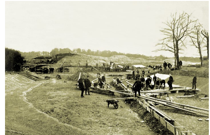
Creating new island excavating and pouring concrete at Heronry Lake -1905. Around 100 unemployed labourers were taken on to do this work, with between 400-500 men being turned away every day. The working day lasted eight hours, from 8am to 5pm with an hour's break for lunch.
