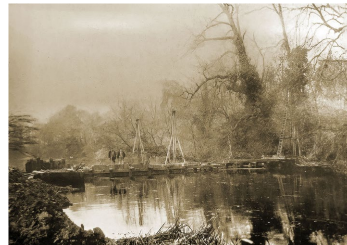
Ornamental Waters Wanstead Park showing piles being driven into the lake bed to construct huge dams isolating part of the Waters for the cleaning scheme in 1909
