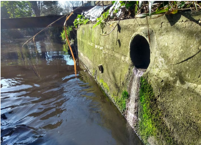
There are countless outlets into the River Roding. They are designed to take clean surface water from adjacent areas into the river and out to sea. However, under certain circumstances raw sewage and other pollutants can end up being discharged into our river. A problem that is becoming more and more frequent due to an ageing infrastructure and greater numbers of homes and other development - pic by Alan James.
